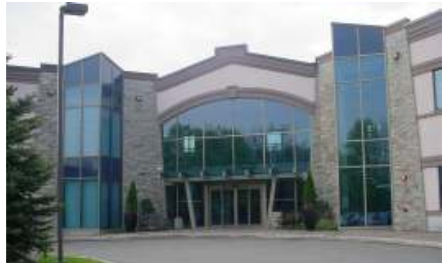
Figure 9: Existing low-rise office building.
