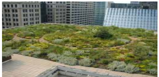
Figure 14: Green roofs ameliorate the urban heat island effect and support natural habitat.
